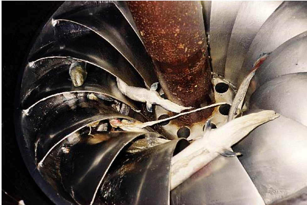
Figure 3.6: A Francis runner clogged with dead fish (Photo: Alex Haro)
